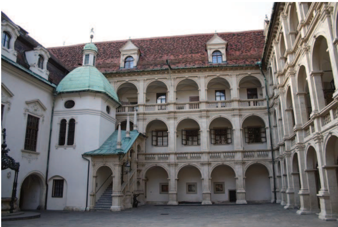
Fig. 8.: The inner courtyard in the Herrengasse 16. building
